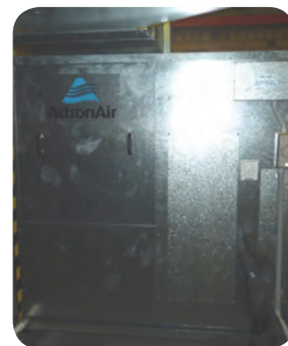
Image (C) INDOOR MODEL: ELY470T-6Q1 Indoor Fan Coil Unit with EC Motor and Plug Fan.
