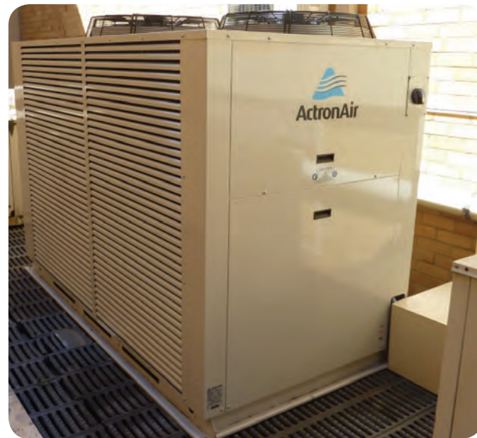
Image (A) OUTDOOR MODEL: CAY470T- 6Q1 (Outdoor Condensing Unit.)
